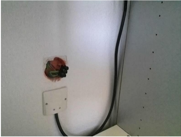
CUISINE-ELECTRICITE et GAZ
